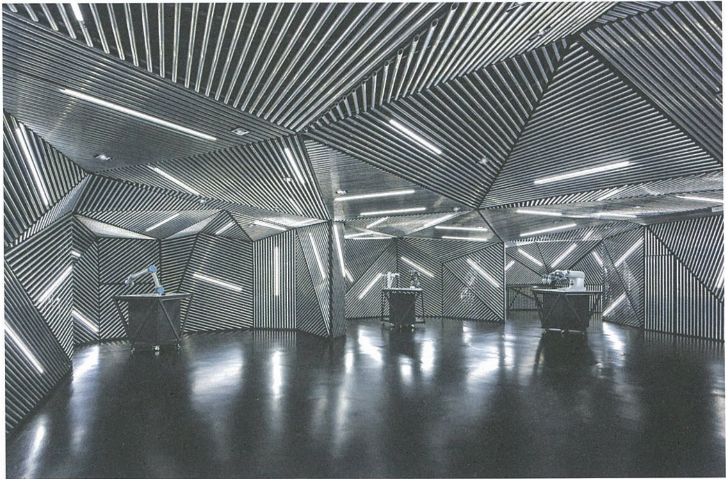
The multifaceted interior walls and ceiling surfaces are layered with 6,000 hollow aluminium tubes and LED lights positioned in an array of angles to create drama against a foil of black
