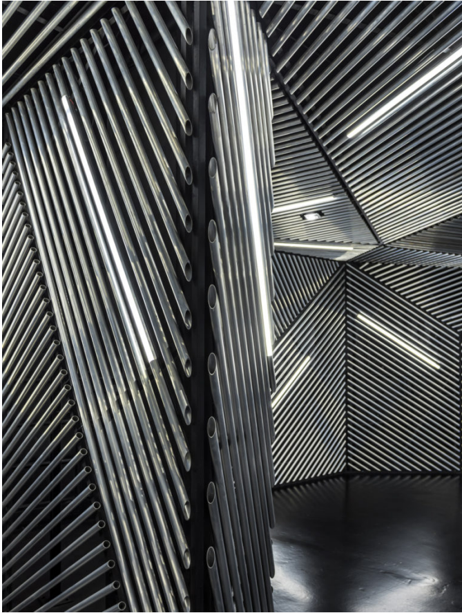
Each facet comprises stacked layers of hand-cut aluminium hollow tubing
